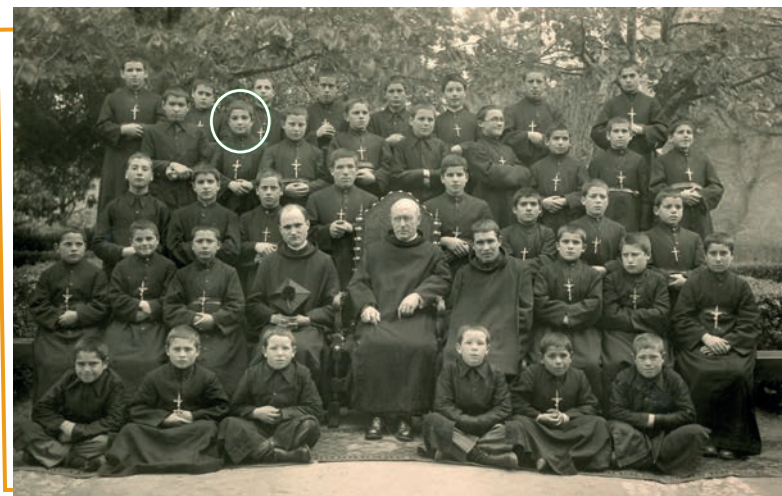
Health Centre at Telhal (Sintra), 1942.
